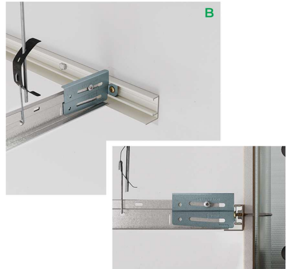
Fig 7. Floating Ceiling-Wall Connection with M90 Clip (see also Fig 12 on Page 10)
