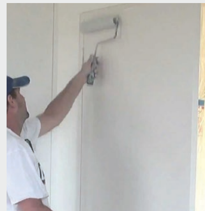
Hung door needs 2 finish coats.
